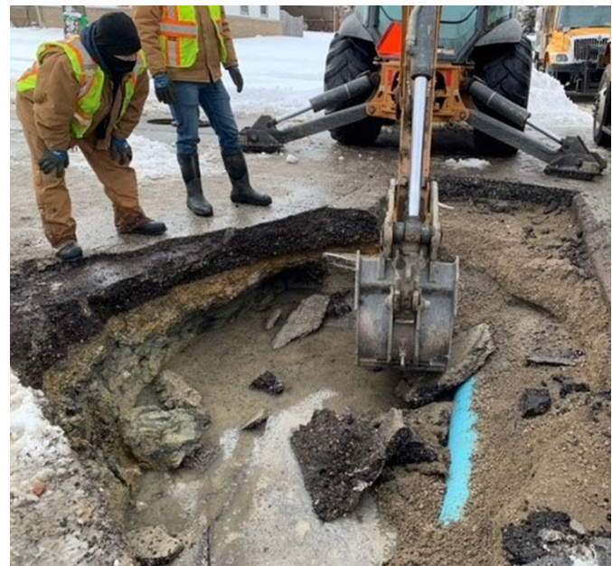
Excavation to repair leak discovered by Aquify's system analysts
