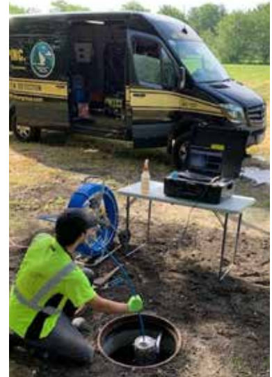
The multiparameter tethered inspection tool is lowered into 12 inch main
